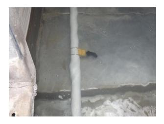
Return piping with directional jets, adjusted to prevent stagnant areas and particle build up in basin.
