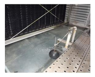
Picture of the cooling tower basin and filter media, conditioned by the system. Scale has dropped off and the water is completely translucent and free of cloudiness. No odors are perceived and no algae growth has been observed anywhere in the tower.
